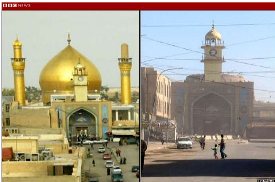
The al-Askari shrine's two minarets collapsed following explosions. The dome of the same mosque, one of the most important sites in Shia Islam, was destroyed in a bombing in 2006, Photo: Getty Images
